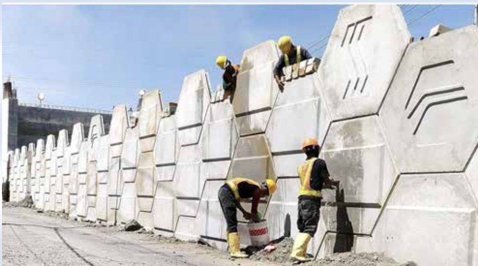
Nehemiah Wall in the Process Of Construction
