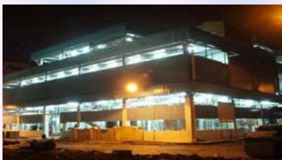
Winter Grade Palm Biodiesel Commercial Plant
