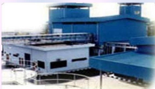
CAROTINO® Commercial Production Plant
