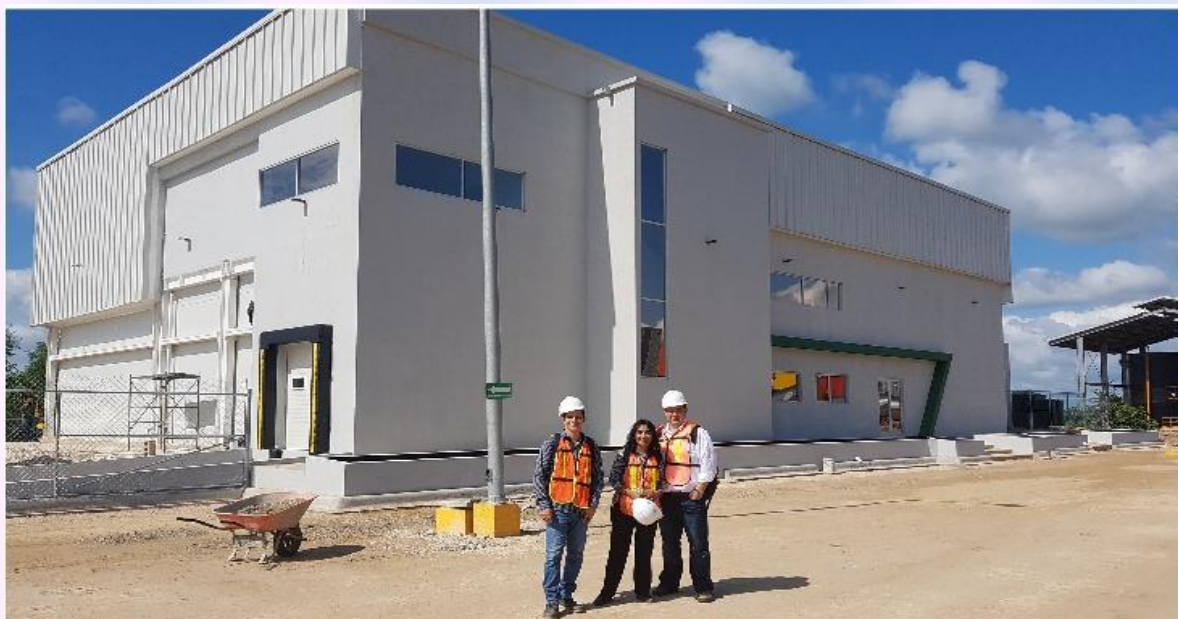
World's first Phenolic Commercial Production Plant in Mexico
